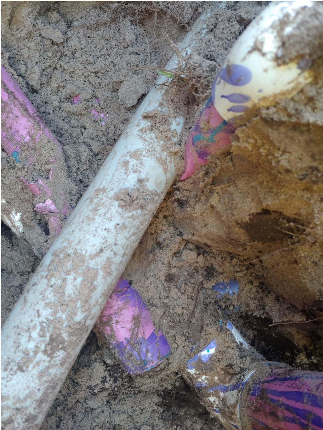
Irrigation zone pipes damaged during directional bore at Paseo Al Mar and Milestone.
